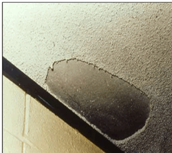
Figure 4 Sprayed asbestos
